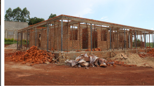
Medical Clinic progress- it is 3,150 sq feet.
