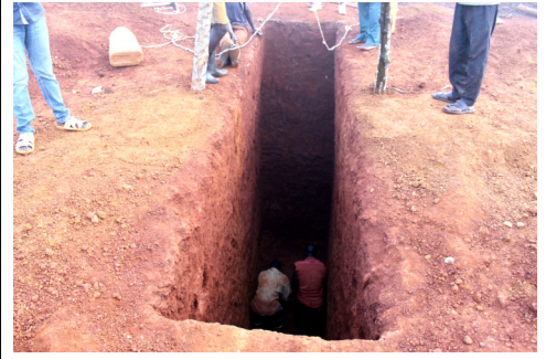
Digging Clinic latrine (see 2 men down in Pit)
